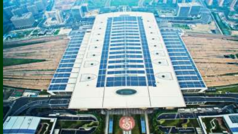
Roof Photovoltaic Power Station of Hangzhou East Railway Station 10MW | Hangzhou, Zhejiang Province, China
