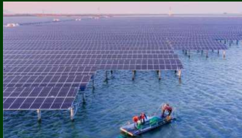
The Largest Fishing-Solar Hybrid Project in Asia 550MW | Wenzhou, Zhejiang Province, China
