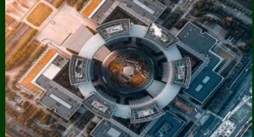
Hangzhou Civic Center Podium Roof Photovoltaic Power Station 1.2MW | Hangzhou, Zhejiang Province, China
